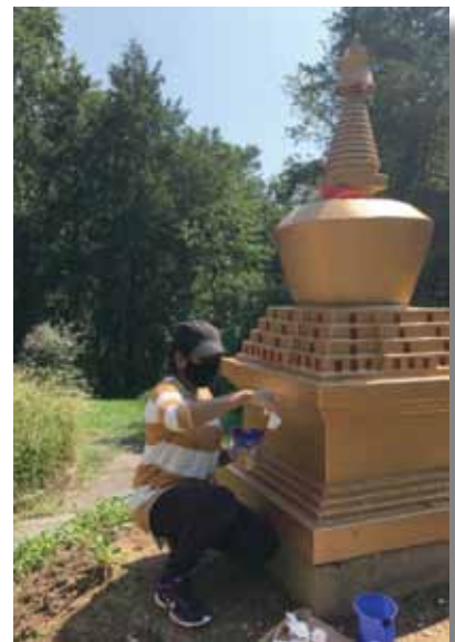
Repairing small stupas at the Palyul Peace Park in Maryland.
