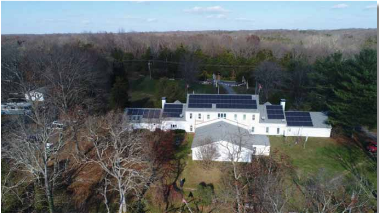
Solar panels were installed on the main temple, a major step in reducing electricity bills as well as feeding solar energy back into the electricity grid. And notice the beautiful fresh paint at the back of the temple!
