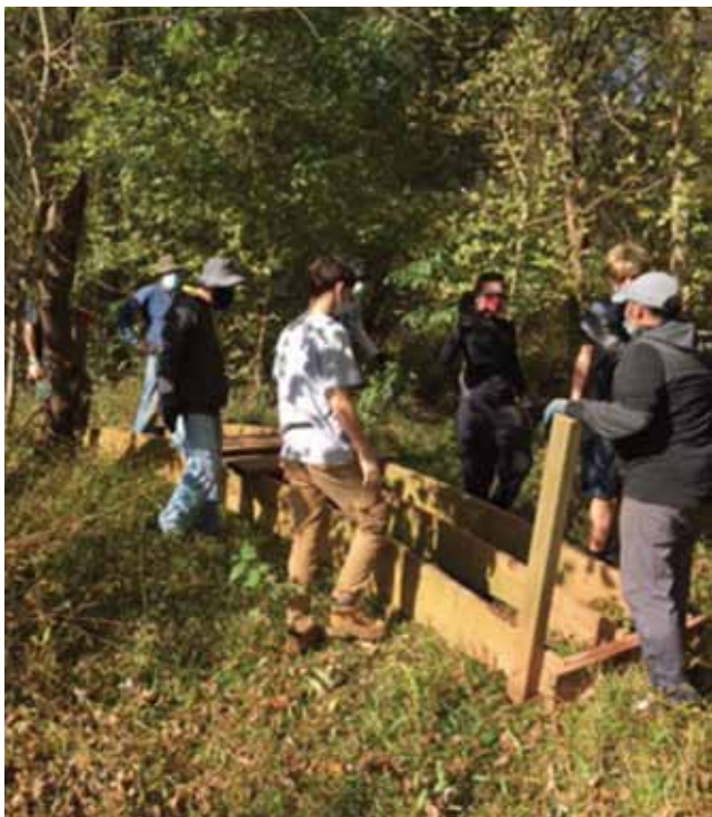
Boy Scouts dismantling a bridge.
