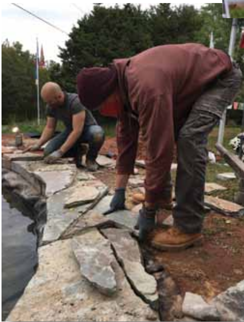
Next steps: completing the fish-pond and laying stone work.
